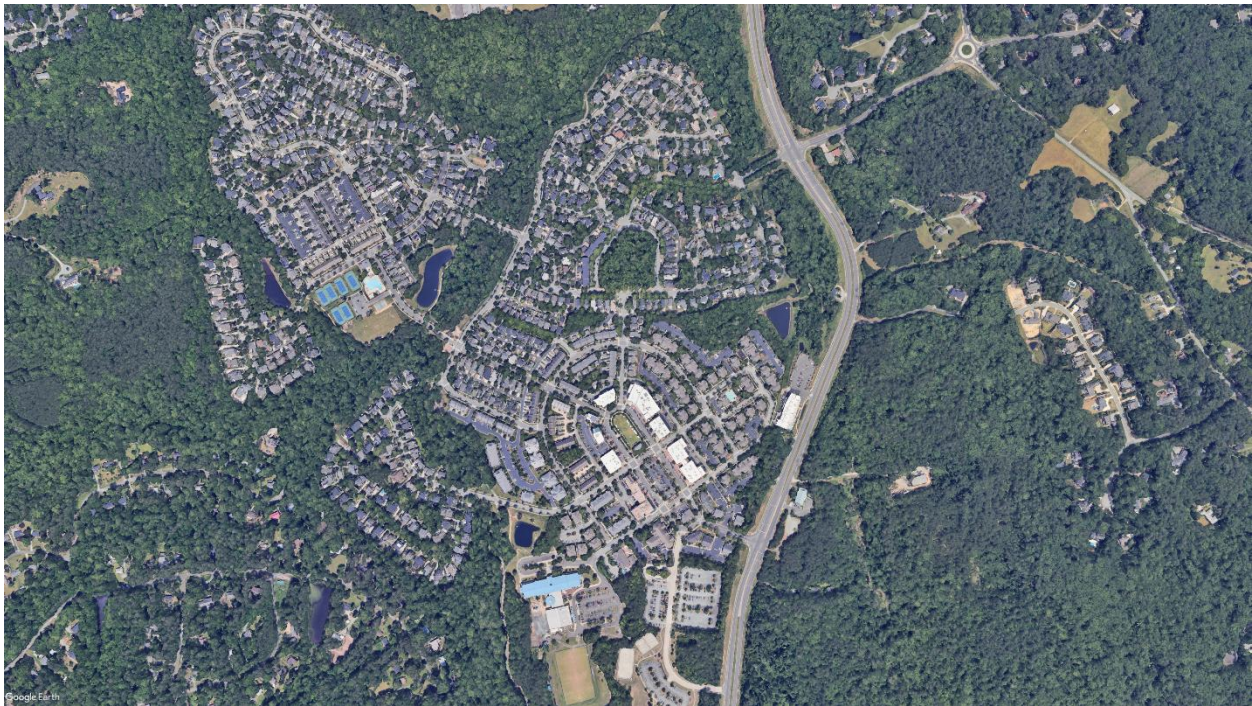
Figure 4. Example of Mixed-Use Center (Aerial of Southern Village, Market St. and U.S. 15-501)
